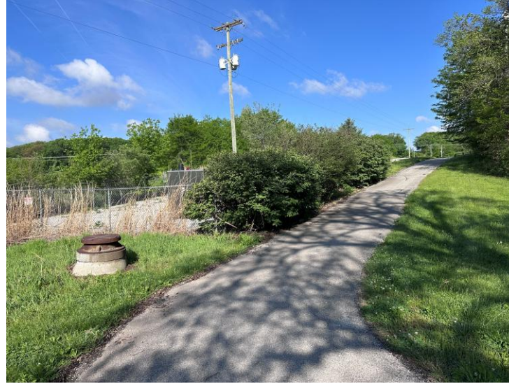
Northeast corner of pump station, looking west
