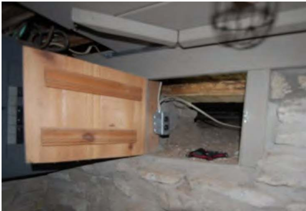
Figure 10. Crawl Space Door that needs weatherstripping. (SRJA 2015)
