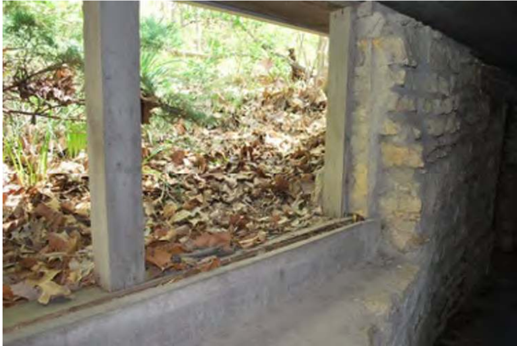
Figure 5. Rear breezeway east wall deteriorated wood framing. (SRJA 2013)
