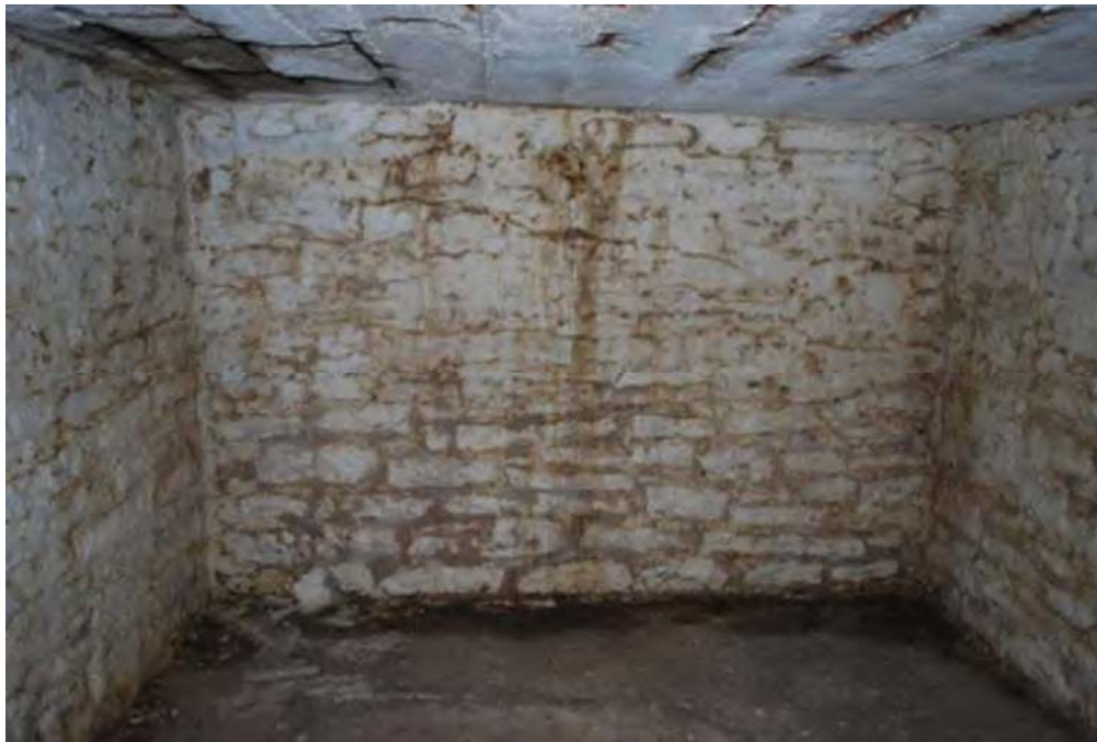
Figure 22. Interior of root cellar. Note the deteriorated steel reinforcing in the concrete ceiling. (SRJA 2013)
