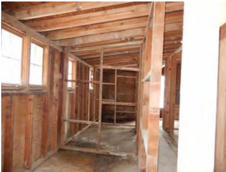
Figure 18. Phase 2 – South Annex: Replace existing moisture damaged wood studs at east wall and deteriorated floor. (SRJA 2013)
