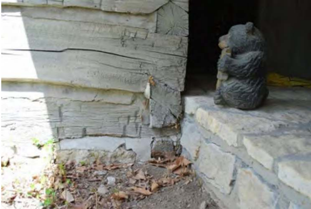
Figure 3. Sill log is buried below grade. The soil needs to be re-graded to at least 6" below the bottom of the sill log. (SRJA 2013)
