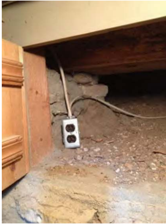
Figure 43: Unsupported receptacle and wiring in the crawl space (WLC 2013)
