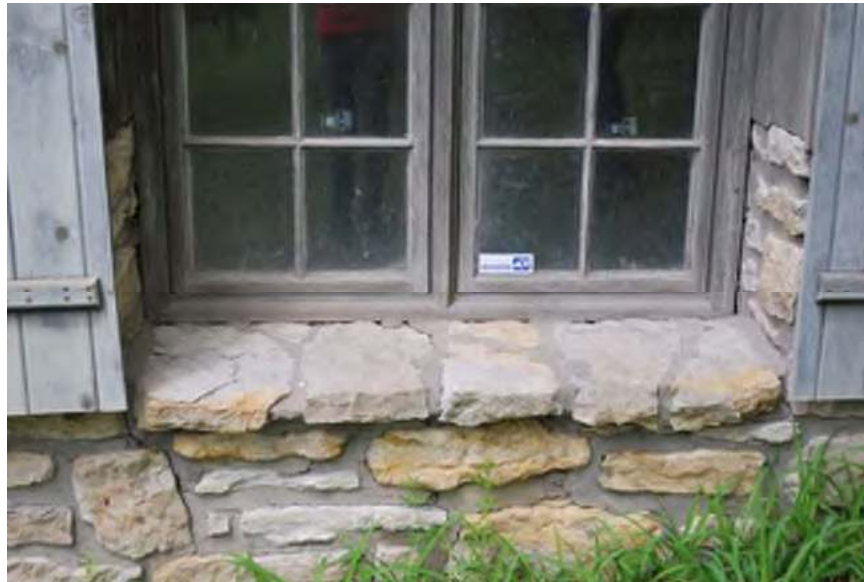
Figure 45. Phase 2 – Annex/Addition: Demo existing stone sill. (SRJA 2013)
