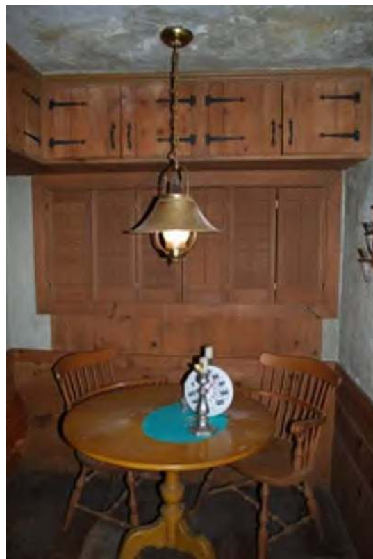
Figure 14. Breakfast Nook: Note the significant plaster damage to the ceiling in this space. (SRJA 2013)
