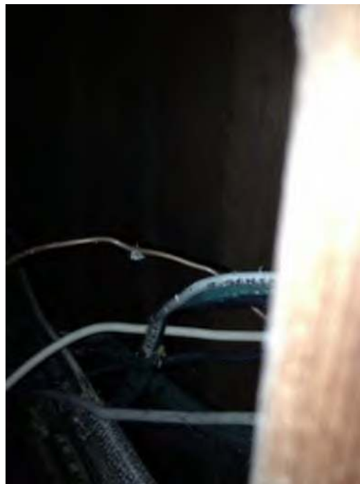
Figure 44: Wiring without protective jacket (WLC 2013)
