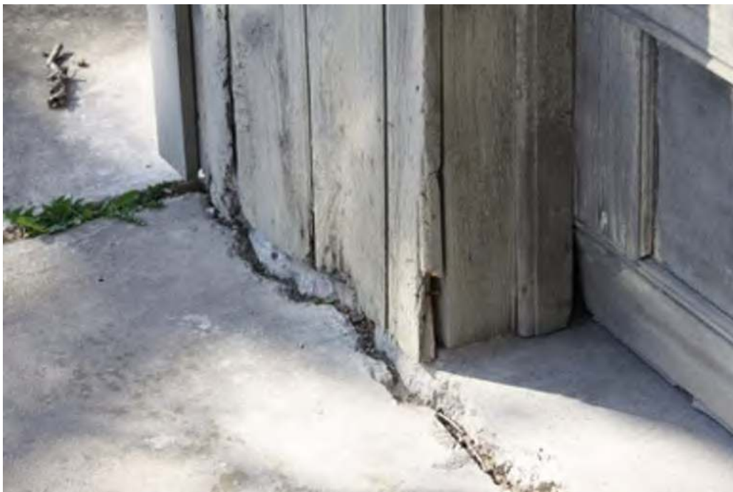
Figure 4. Detail of deteriorated garage trim and open cracks in the concrete drive. (SRJA 2013)
