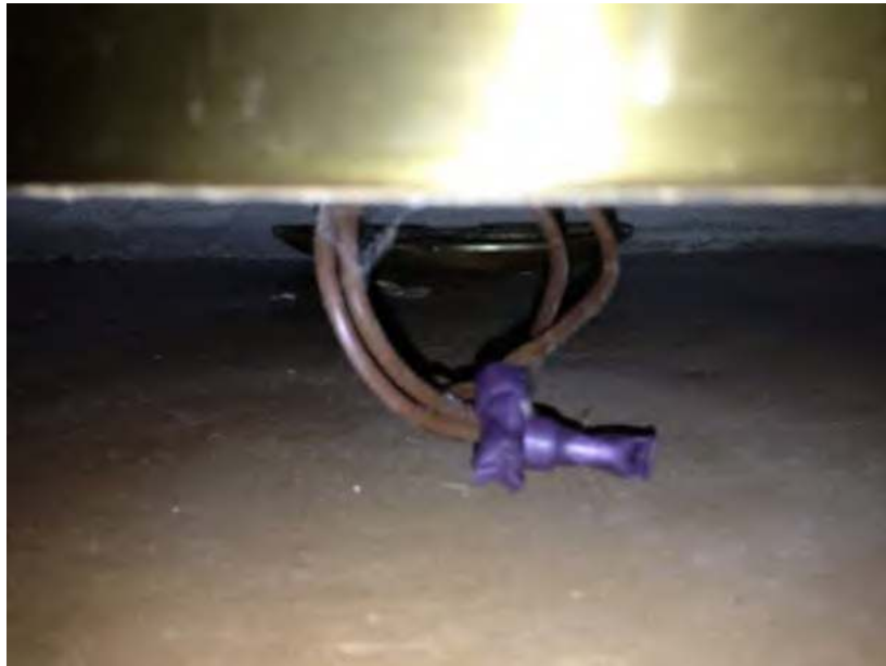
Figure 41: Wiring connections below a lamp (WLC 2013)
