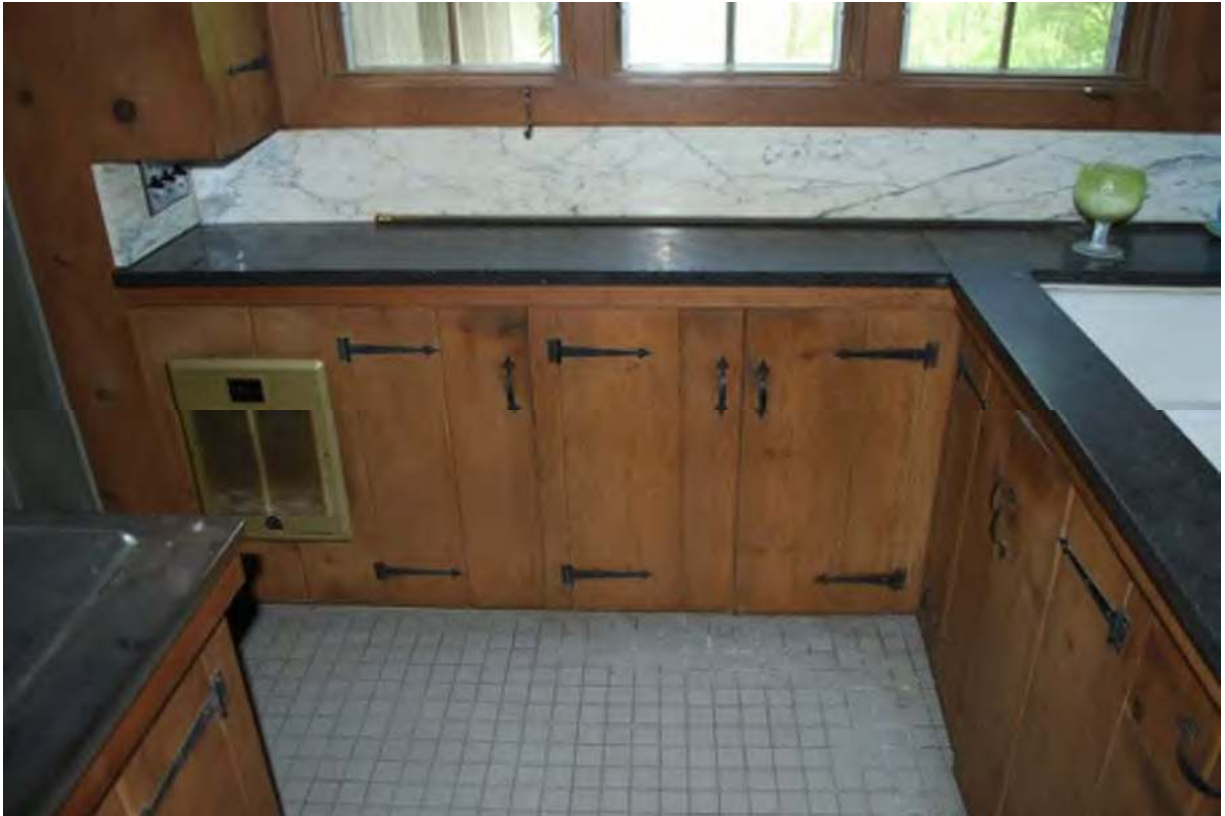
Figure 15. Kitchen: Clean existing tile floor and re-grout where necessary. (SRJA 2013)
