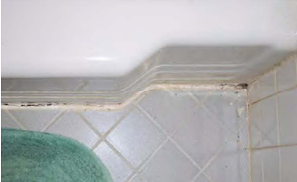
Figure 13. Bathroom 105: Bathroom grout and caulking deterioration. (SRJA 2013)
