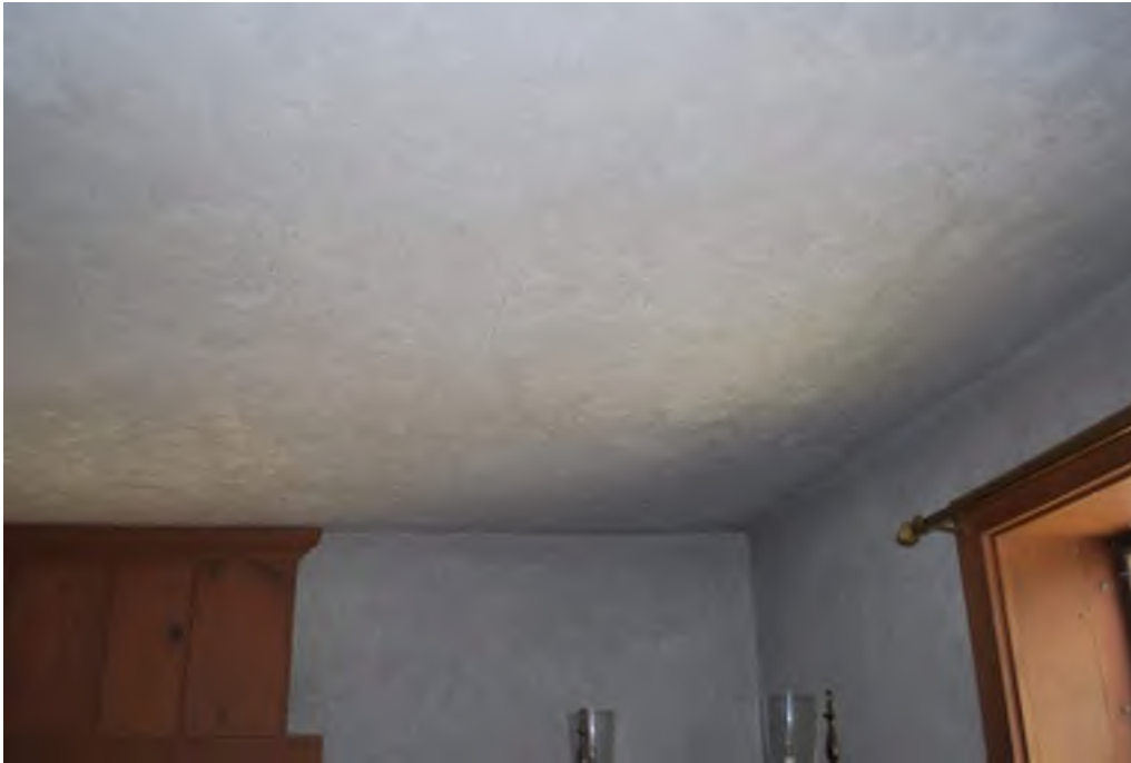
Figure 11. Living Room 106: Damaged plastered ceiling. (SRJA 2015)
