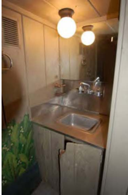
Figure 9. Bathroom 003: Damaged wood cabinet door and stainless steel counter. (SRJA 2015)
