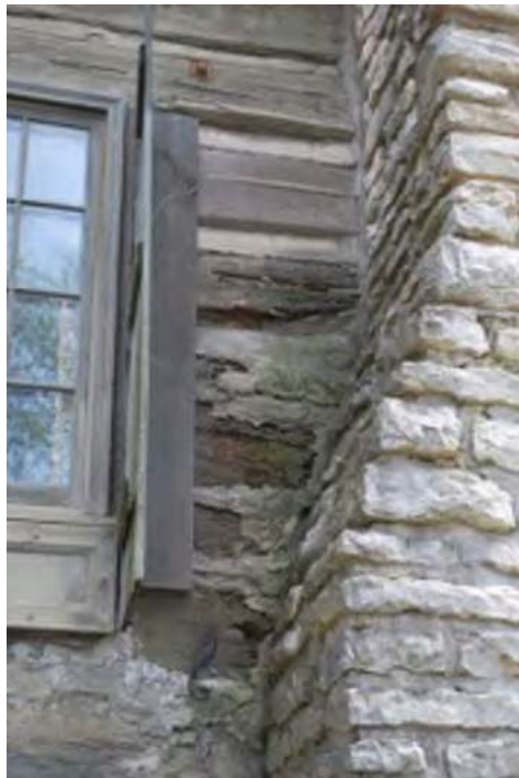
Figure 2. Detail of the deteriorated logs on the west wall adjacent to the stone chimney. This is due to poor construction detailing as the stone chimney abuts the logs, west elevation. (SRJA 2014)
