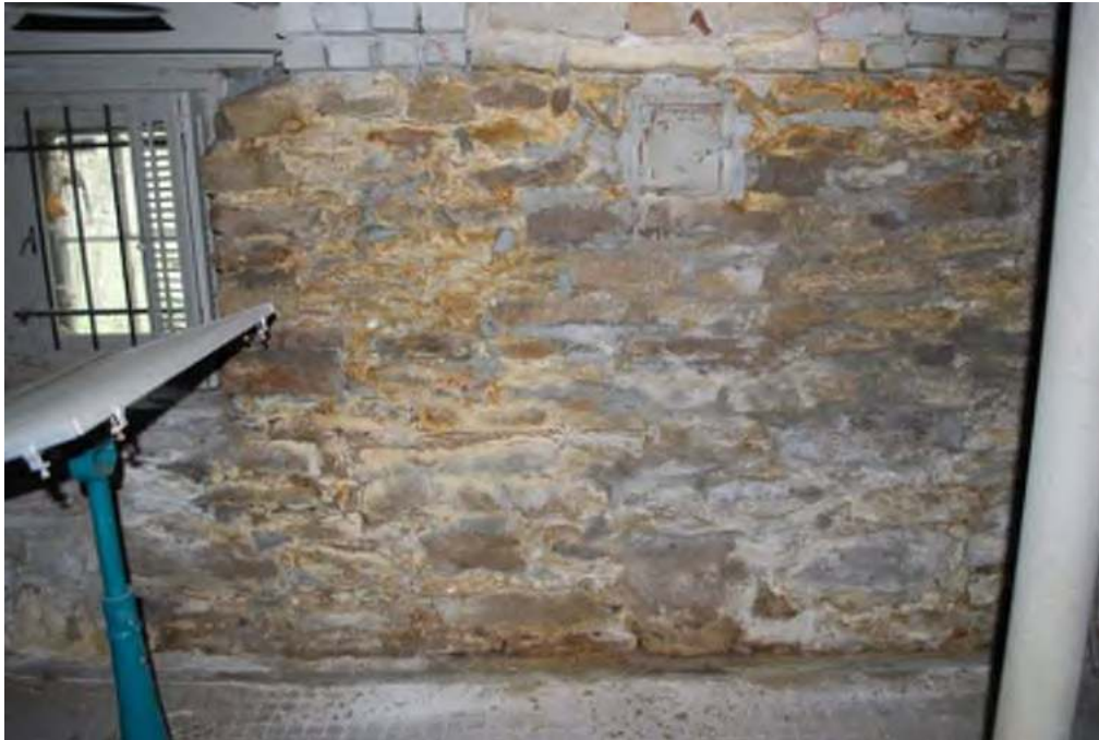
Figure 7. West stone foundation wall in Basement Room 001 to be thoroughly cleaned. (SRJA 2013)
