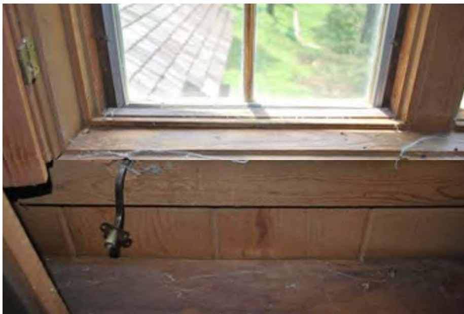
Figure 16. Second Floor: The casement window crank cover has become unattached and needs to be reattached with longer brass screws. (SRJA 2013)
