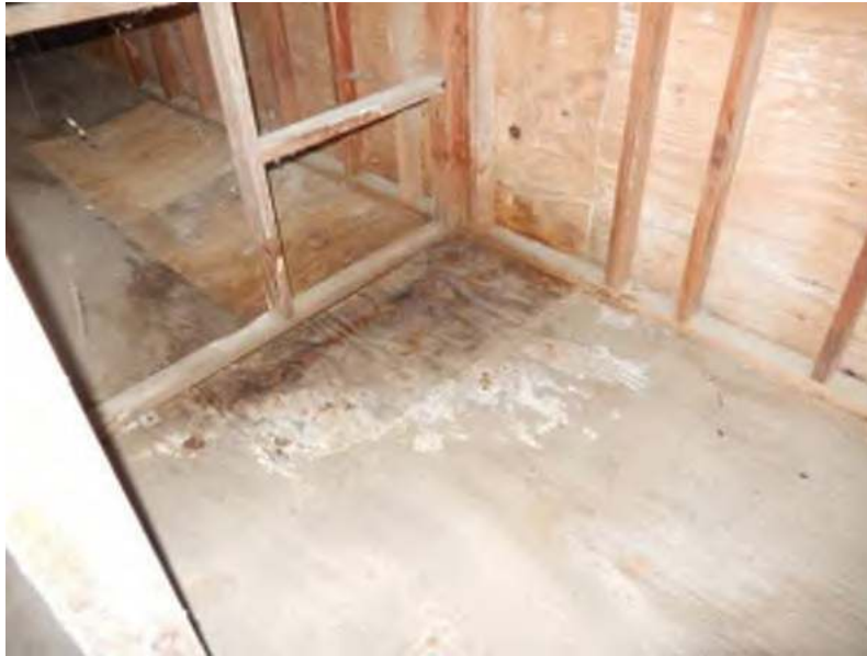
Figure 23: Deteriorated framing and subfloor at the east wall of the South Annex. (SRJA 2015)
