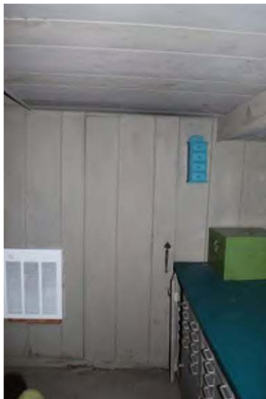
Figure 8. Deteriorated wood partition wall – Door to the storage room that does not fully open. (SRJA 2013)
