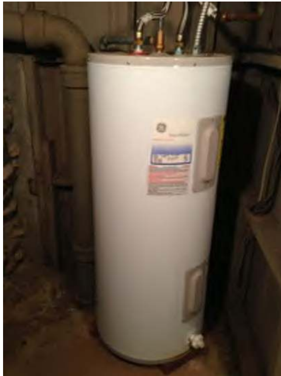
Figure 25: Existing electric tank water heater to be removed. (WLC 2015)
