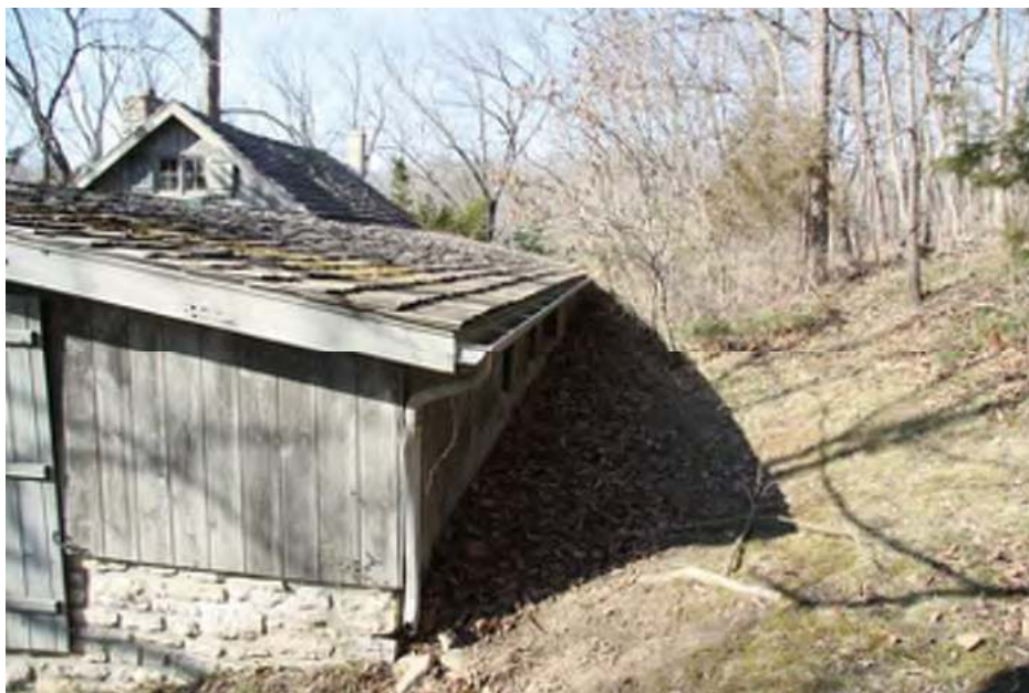
Figure 24. East elevation of the South Annex. This area requires re-grading and new sub-grade drainage. The gutter needs to be repaired and a volunteer tree growing between the gutter and the roof needs to be removed. (SRJA 2013)
