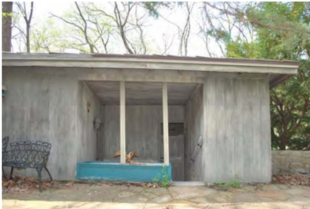
Figure 6. Rear stone patio & east covered porch. Note the wood planter box is deteriorated. (SRJA 2013)
