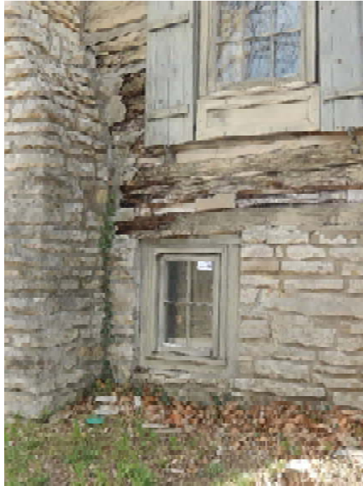
Figure 19: A portion of the rotten log framing on the west elevation of the residence (SRJA 2015)
