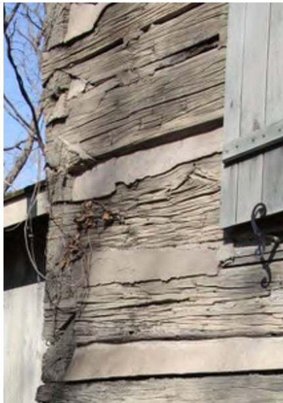
Figure 20: Existing Portland cement daubing (SRJA 2015)
